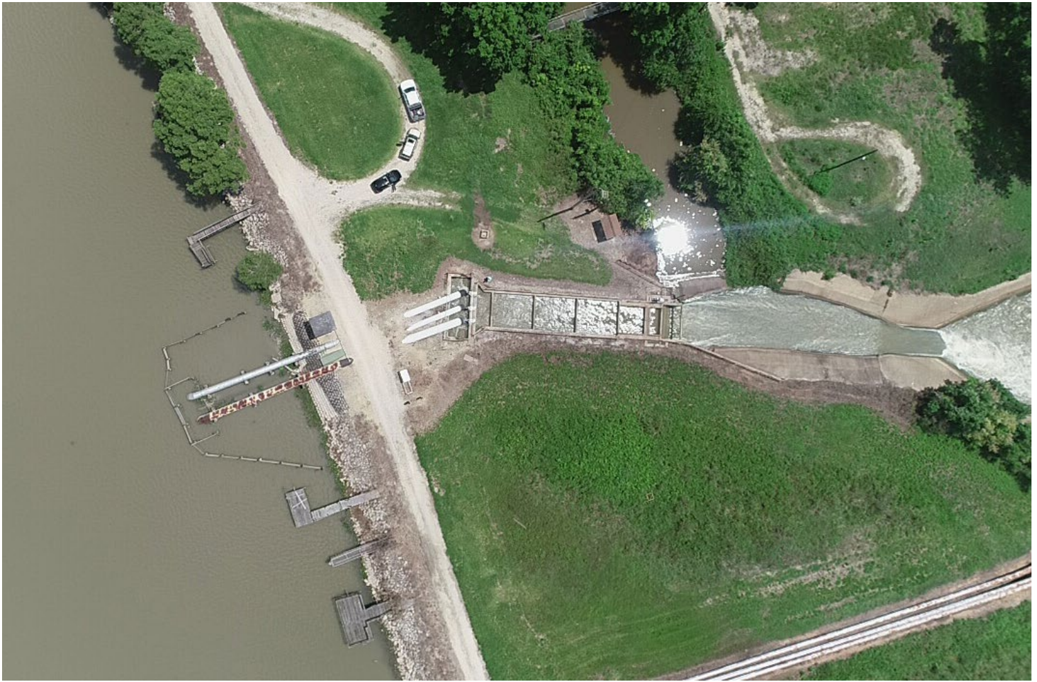
Existing Harris Reservoir Outfall
